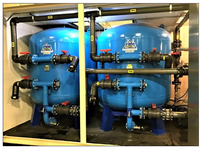
PRM constructed a multi-faceted, comprehensive Groundwater Treatment system. This system is equipped with two inlets, a Gravity Fed linet and a Vault Pump inlet, dual AMT 3152-98 OWS (Oil Water Separator) Pumps, and two Air Strippers (AST). Each AST unit has an Ametek EN 909 Series AST Blower. The system is equipped with access ports above the OWS Tank and both Carbon Vessels.
