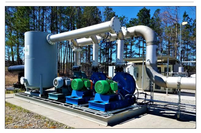
Prm provided a landfill extraction blower system upgrade per Clients RFQ and project manual. Two additional LFG blowers were added to the existing skid unit onsite. PRM provided Variable Frequency Drives (VFD) for each new blower motor along with a new control panel for complete system operations.
