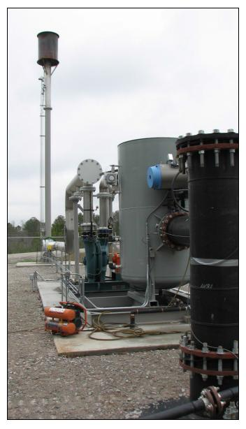
This methane extraction and condensate removal system consisted of a 60 HP gas extraction blower and 3500 SCFM candlestick flare that was designed and manufactured by PRM. Includes a full SCADA control panel package with integrated PLC. The system provides gas to a 6MW generator plant using 24 packages engines. PRM provided system manufacturing, integration, installation, and startup. In 2017 the system was upgraded to include two more 60HP blowers to increase production for the client.
