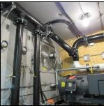
This SVE/AS system was housed in two 8' x 40' Connex containers. One enclosure housed the SVE systems and three Rotary claw compressors. This enclosure was rated for a Class I Div 2 location. The second enclosure housed two Rotary screw compressors and air dryers. This enclosure included a closed off room that contained the main breaker panel and controls.
